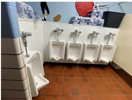
Urinals have new flush valves
