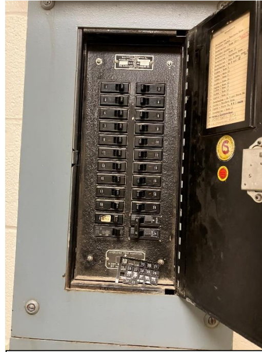
Electrical subpanel
