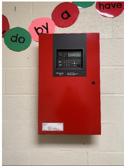
Fire alarm control panel
