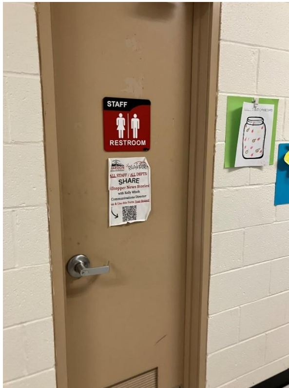
Doors retrofitted with ADA hardware
