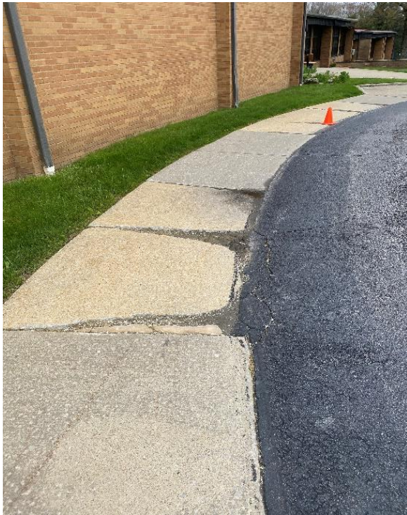
Sidewalk cracking
