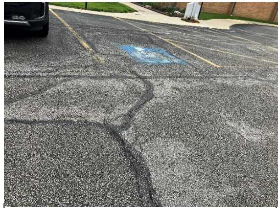
Asphalt in need of resurfacing
